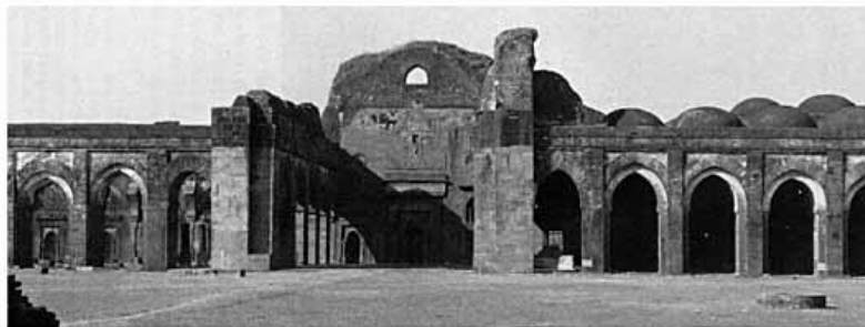
Fig. 6. Interior of Adina Mosque, Pandua (1375). Interior facing western wall, showing collapsed barrel vault. Photo by Catherine Asher.
