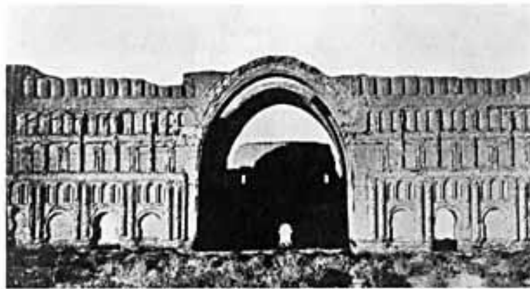
Fig. 8. Taq-i Kisra, Ctesiphon (near Baghdad, third century A.D.). Façade in the late nineteenth century. From Arthur Upham Pope, A Survey of Persian Art (Ashiya, Japan: Jay Glück, 1964), vol. 7, pl. 149. Reprinted by permission of Jay Glück.
